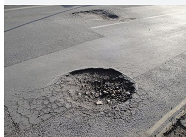
Figure 2: Pothole
